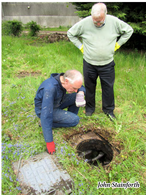
Francis Whitehead and Bob Rowe contemplate one of many mystery manholes uncovered in the area behind the bungalow.
